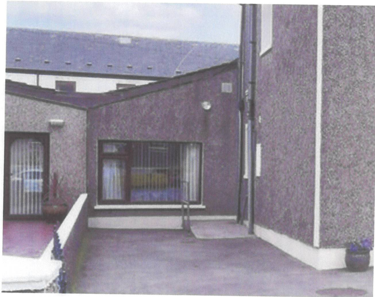
Front View 36 Deanwood Avenue, Togher Cork T12 TRK2
