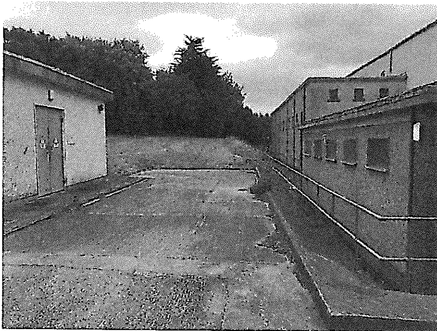
Image 5 The MV building on the left, and the control room building on the right, with the taller 38kV station building immediately to the rear and the dominant 110kV building in the background
