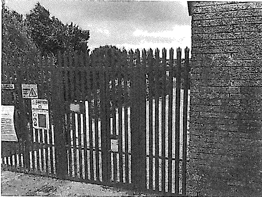
Image 2 The existing entrance gate into Trabeg 110 kV Substation
