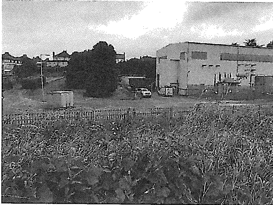
Image 4 View into the site from the grassed area along the Trabeg River, located just outside the southern boundary with proposed development Site A in the foreground, the 110 kV building and associated electrical plant on the right and the internal service road on the left
