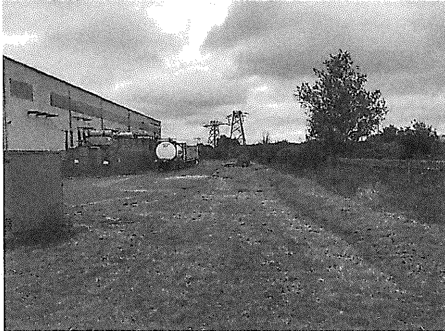
Image 7 View of proposed development site A – showing the 110kV and associated plant on the left, the OHL structures in the background and the existing boundary fence on the right
