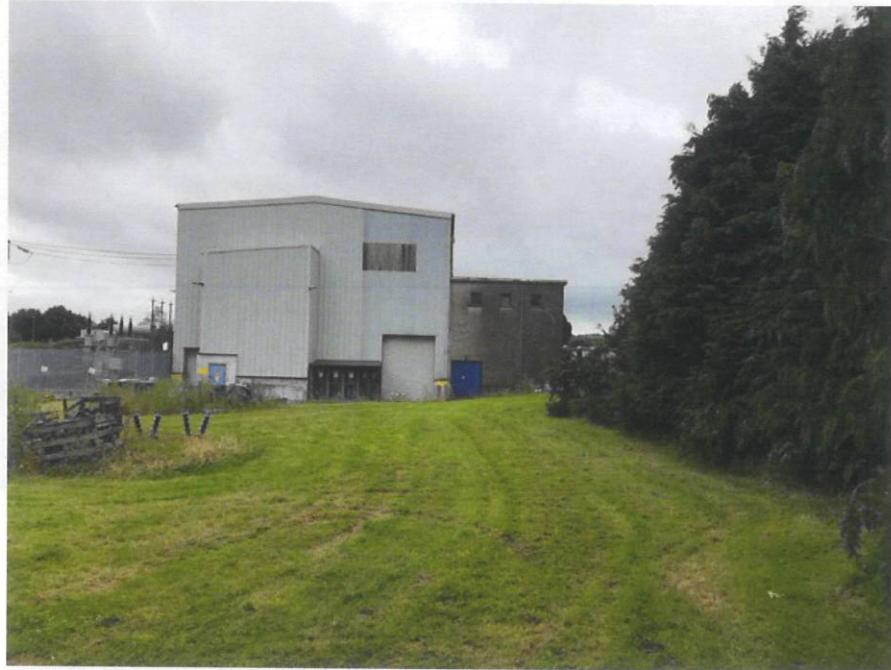
Image 9 View of proposed development site B – facing towards the gable ends of the existing 110 kV and 38 kV substation buildings, with thick band of planting on the right-hand side, which screen the existing buildings from view
