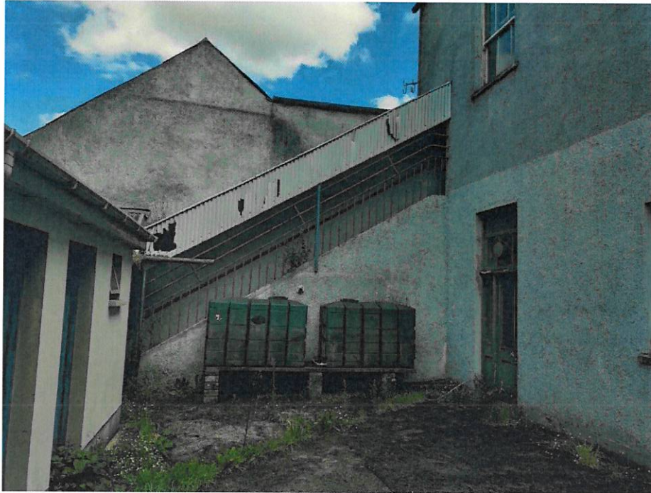
Courtyard First Floor Access to the west.
