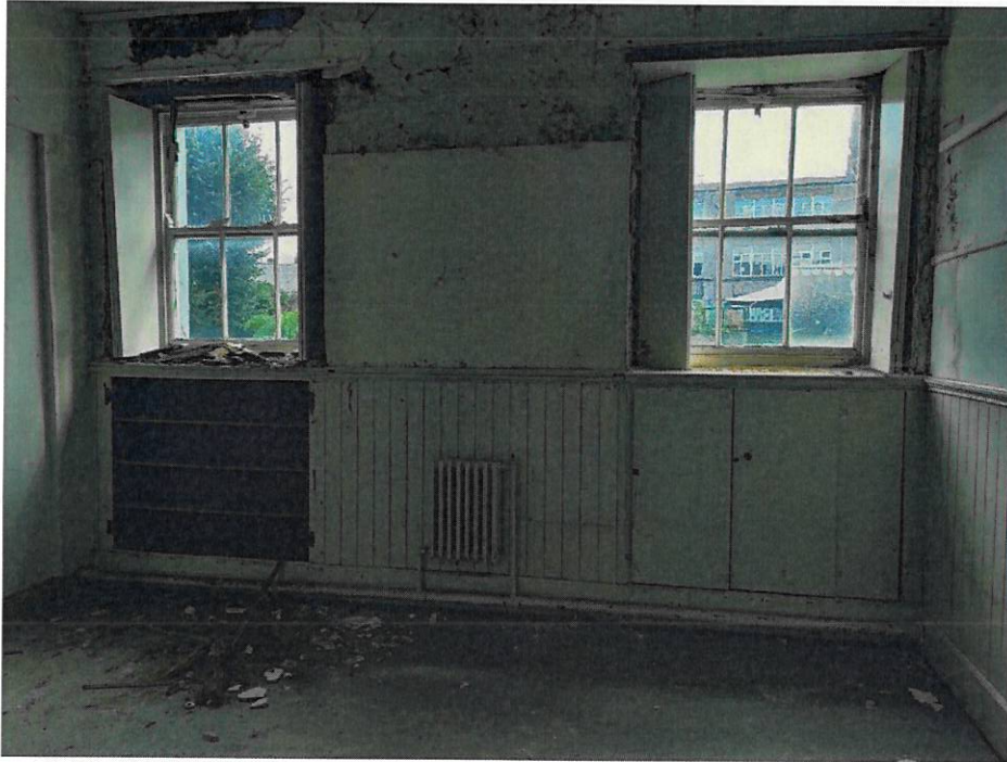
Ground floor room, window detail and wainscoting.
