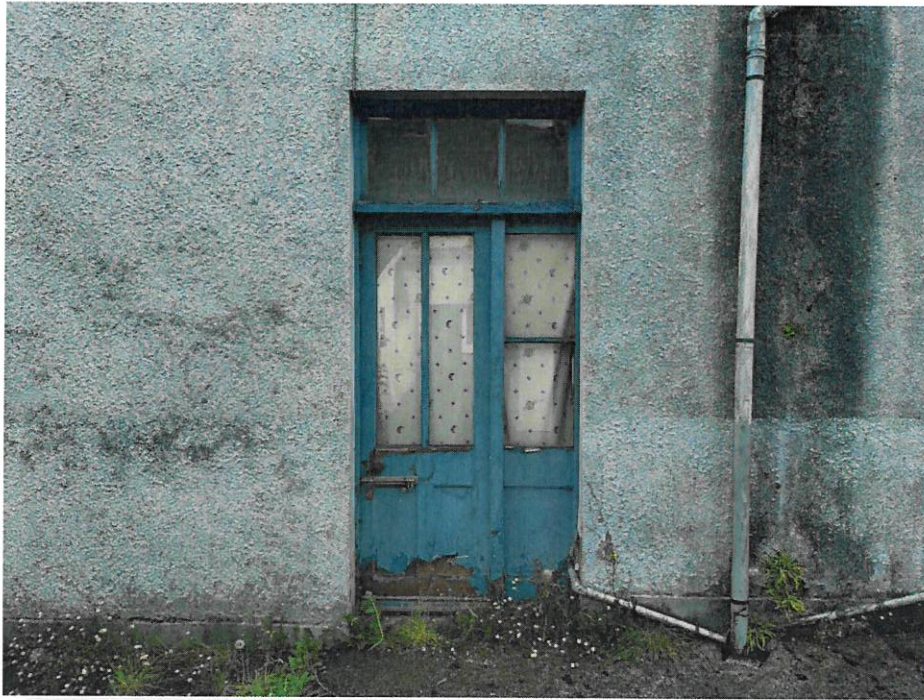
Entrance Courtyard, north elevation historic timber door, blue.
