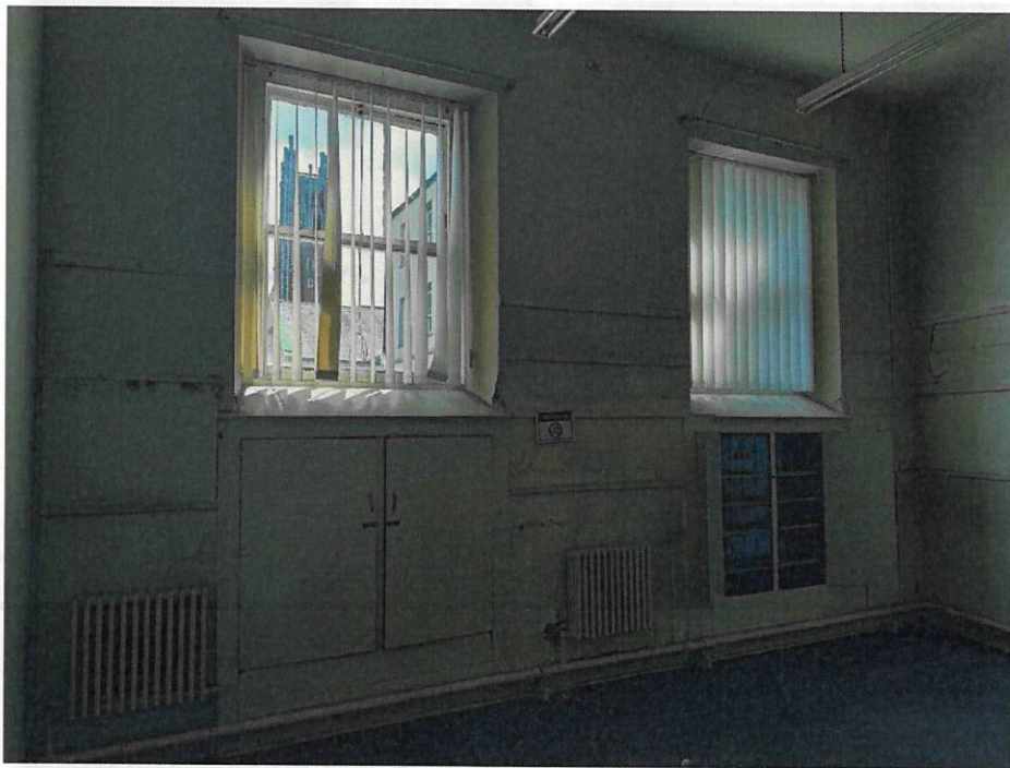
Ground floor room window detail to the south.
