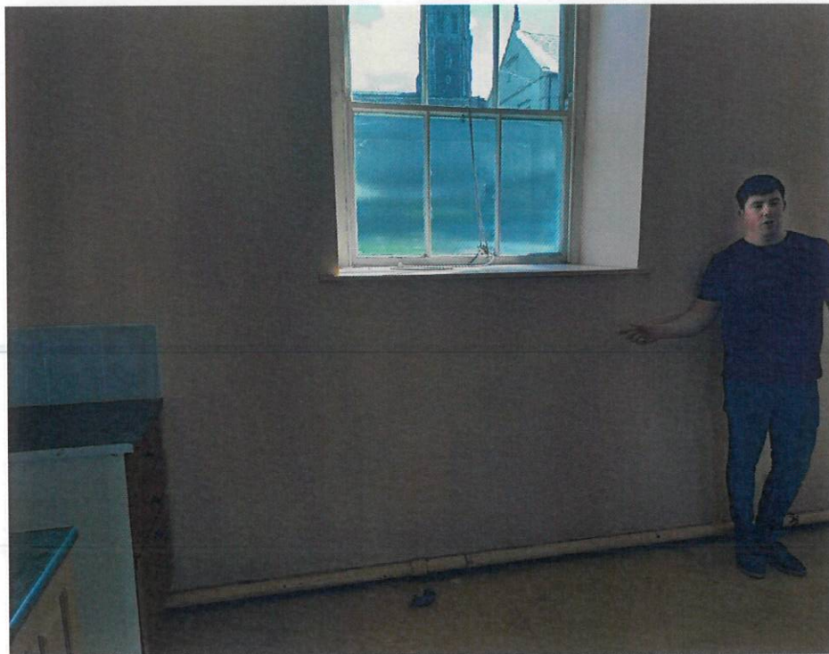
Ground floor room south wall dry lined in plasterboard.
