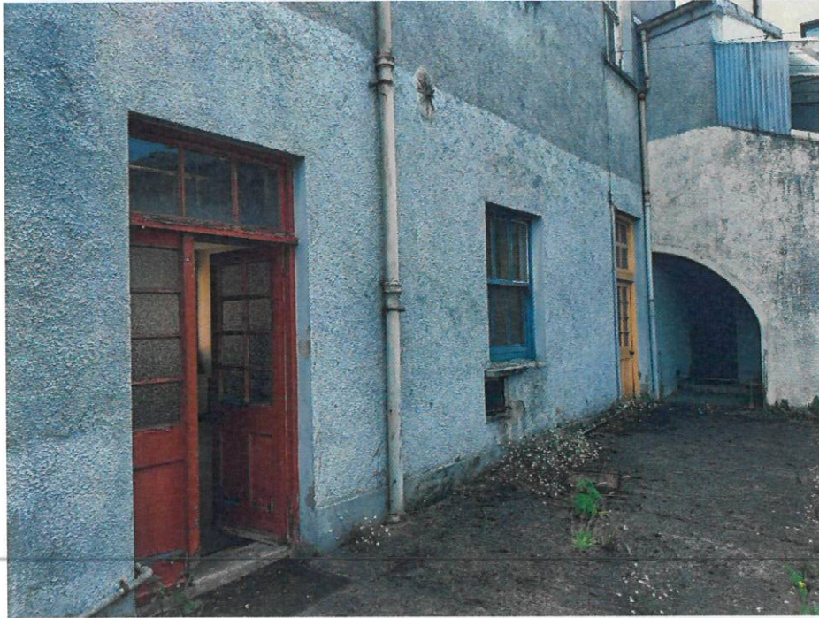
Entrance Courtyard at ground floor, west side, north elevation
