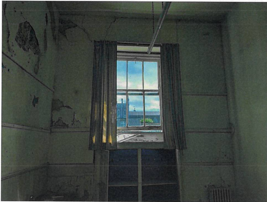
First Floor Room window detail to the south.
