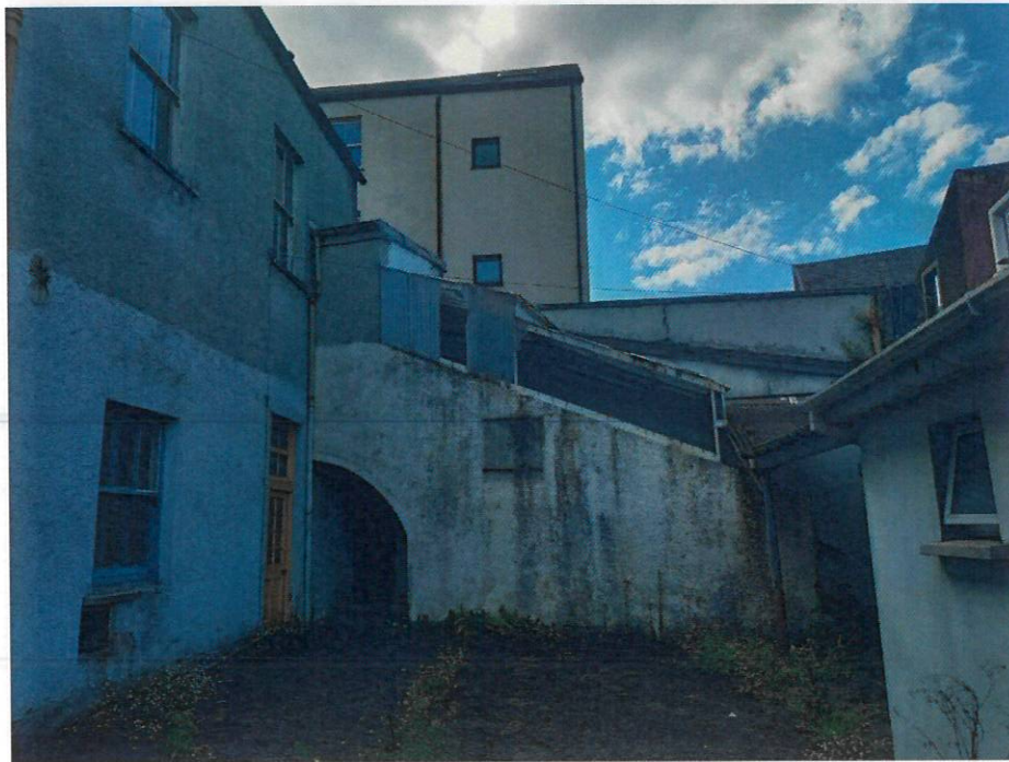
Courtyard first floor access to the west.
