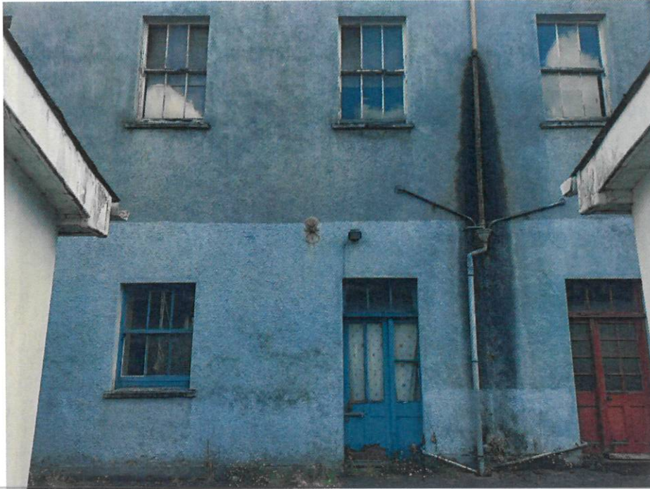
Entrance courtyard view from doorway at Hillgrove Lane.
