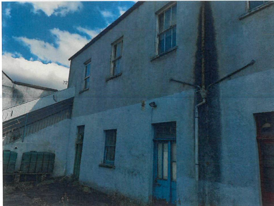
Entrance Courtyard, ground floor east side, north elevation.
