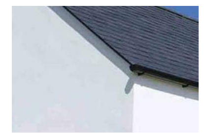
Flush eaves with half round gutter
