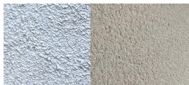
Existing roughcast render contrasting with proposed new smooth render for sections of new construction.
