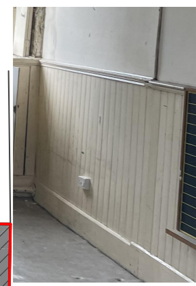
Existing wall panelling
