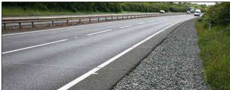
Figure 5.9: Roadside Filter Drain
