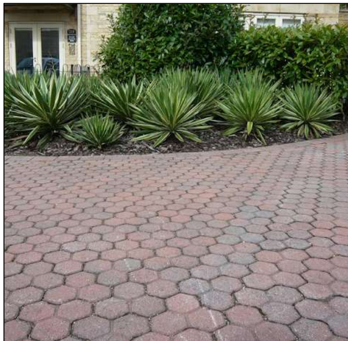
Figure 5.3 Pervious Pavement ( www.susdrain.org )
