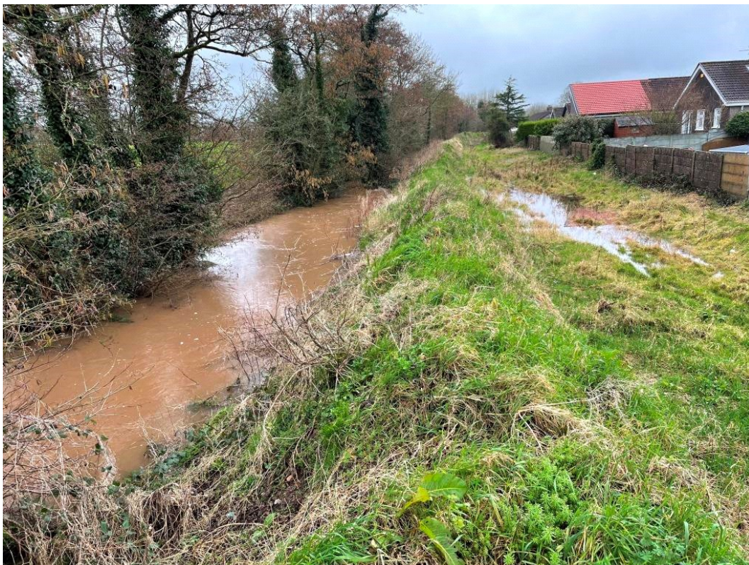
Photo 12: Maglin North, downstream of Maglin Road Bridge
