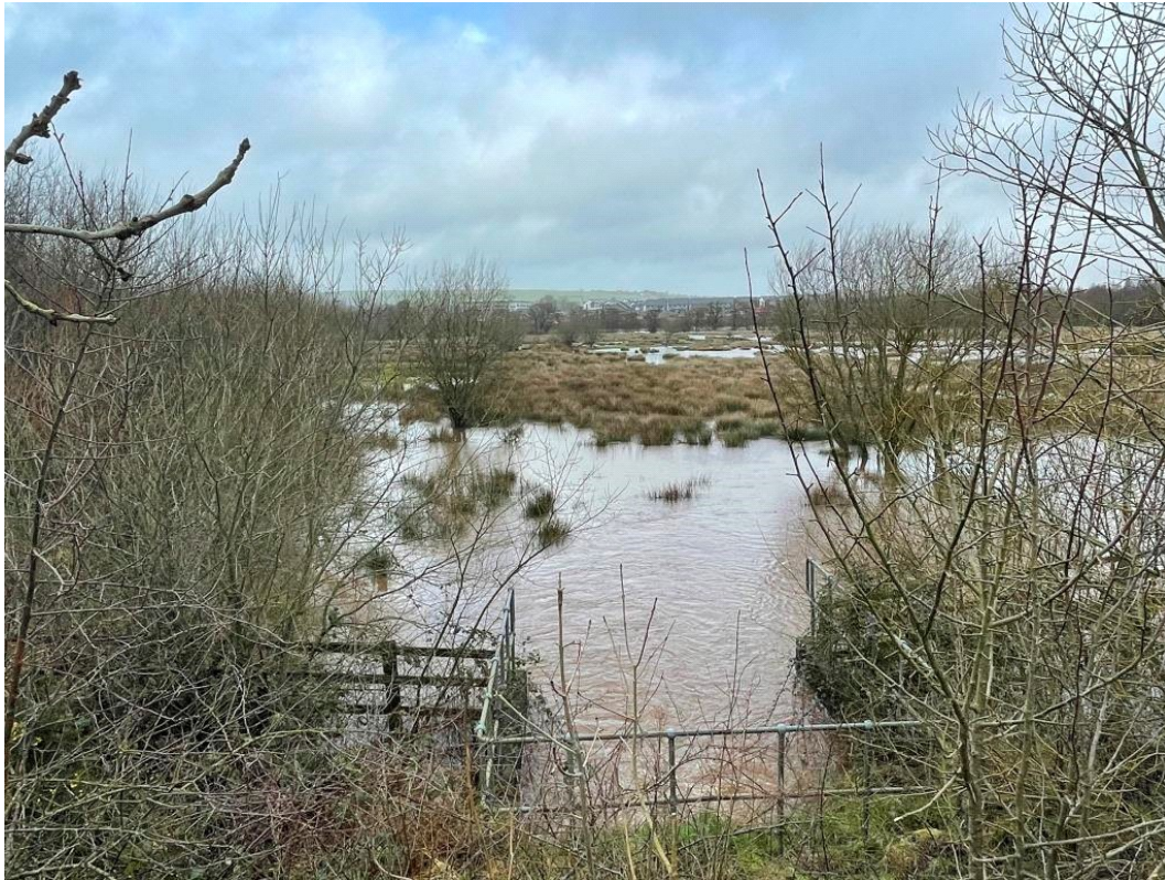
Photo 13: Twin pipe culvert under N22 linking Maglin South with Maglin North
