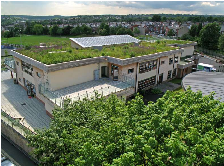
Figure 5.4 Green Roof ( www.bauder.co.uk )
