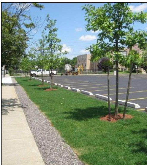
Figure 5.6: Infiltration Trench
