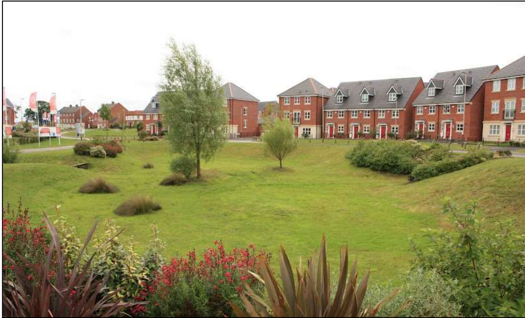
Figure 5.14: Detention Basin ( www.susdrain.org )
