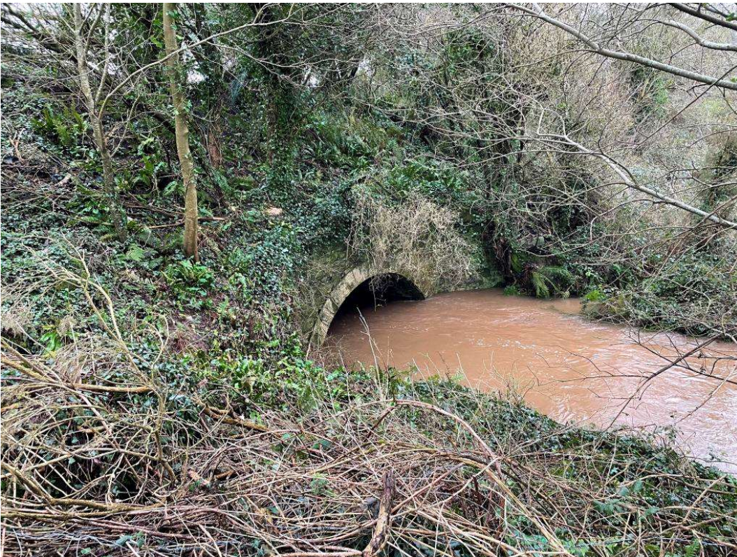
Photo 16: Clash Road Bridge, upstream
