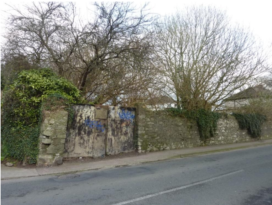
Site at South Douglas Road
