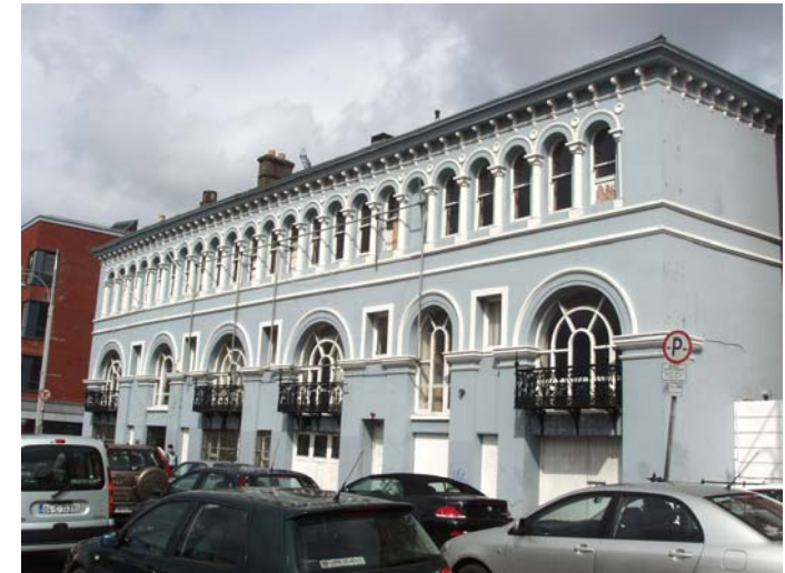
Three-storey building fronting onto river
