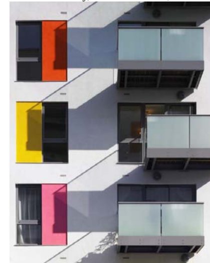
Subtle use of colour at Abbots Wharf, Tower Hamlets, London
