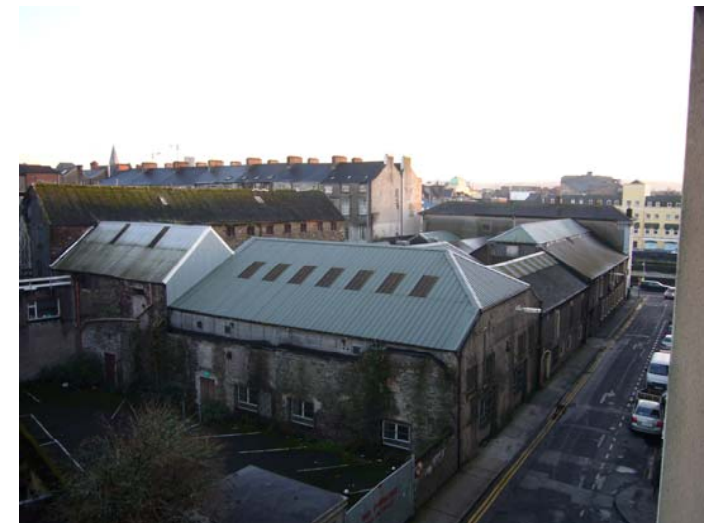
Complex of warehouses located to the rear
