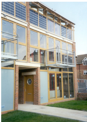
Solar Panels- Bedzed, Surrey
