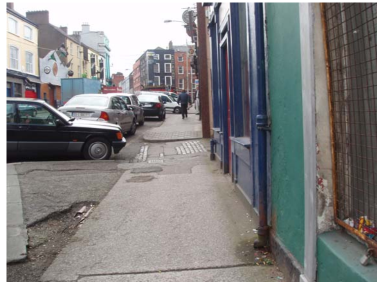
Coburg Street- poor quality paving and haphazard parking
