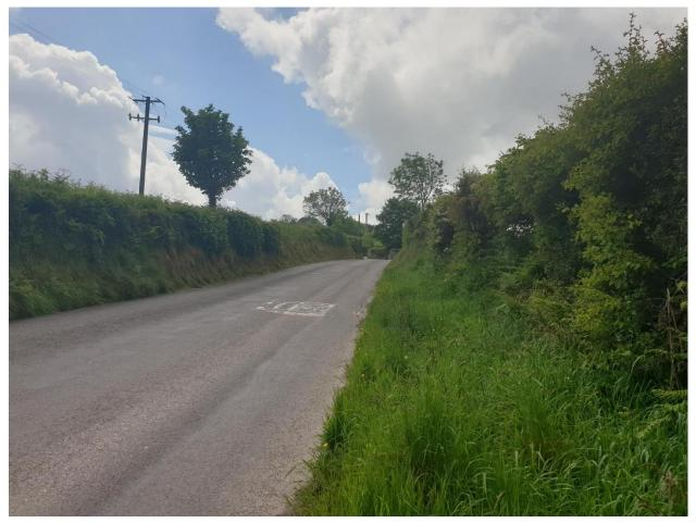
The posted speed limit on both the Lehenaghmore Road (L2455) and Togher Road (L2454), within the scheme extents, is 50kph. The existing horizontal and vertical alignment does not comply with standards. Several side roads do not have 'dwell areas' where they meet the local road.
