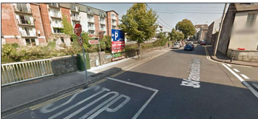
Figure 29: View of existing defences at Crawford Hall
