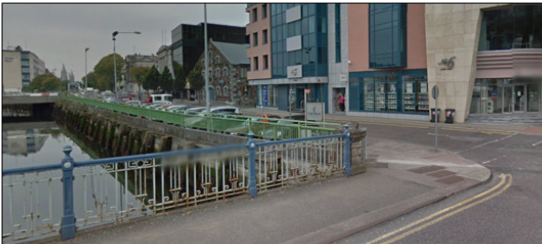
Figure 31: View of Lapps Quay West at St Vincent's Bridge from Clontarf Bridge
