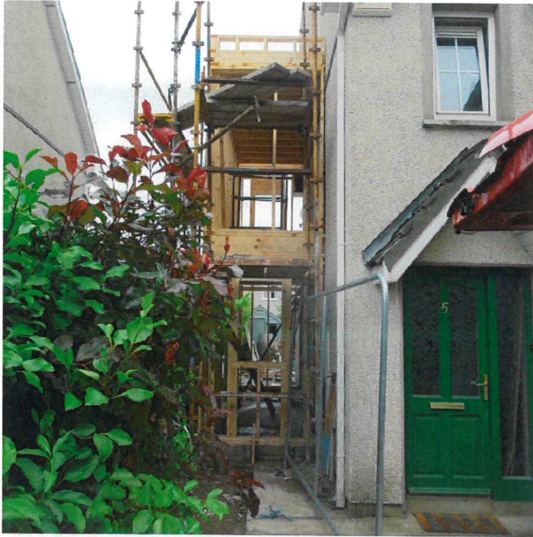
Front elevation with extension to side under construction
