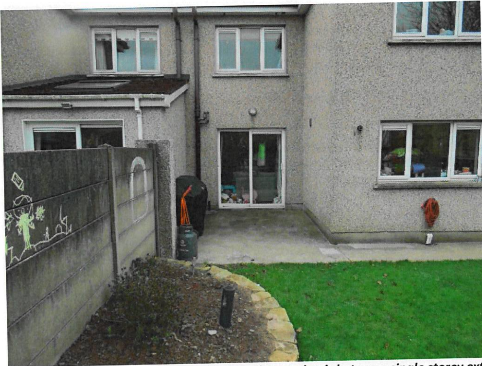
View of north elevation of house. Proposed extension is between single storey extension on adjoining property to left and two storey annex of house
