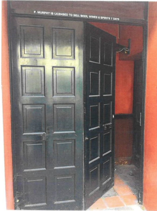
Image of existing bar door
