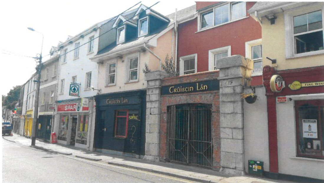
Existing Front View of Bar Entrance including Protected Structure 'Stone Archway to Former St. John's Market'
