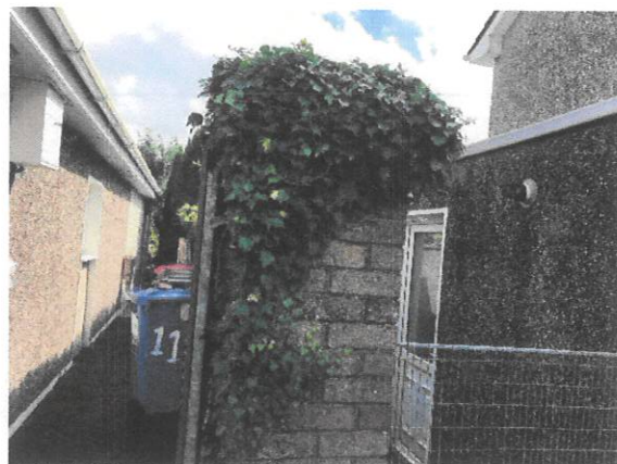
View of Side Passage from Front
