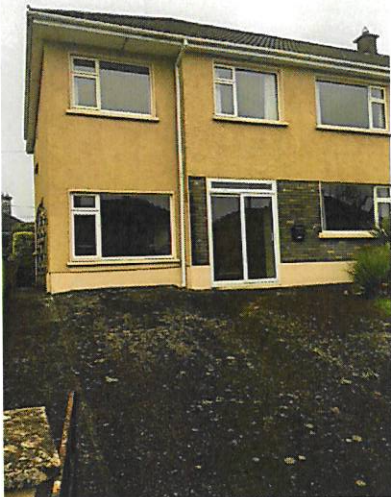
Front elevation of dwelling
