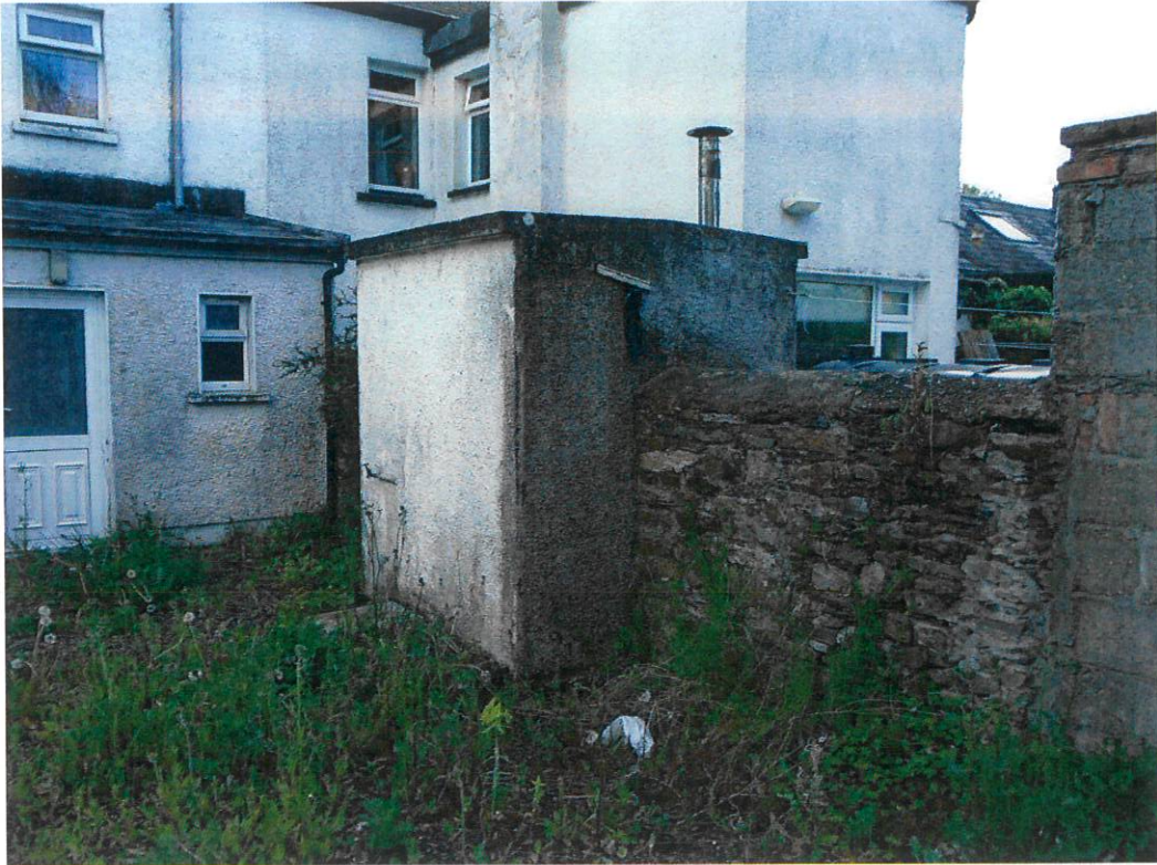
EXISTING TOILET ENCLOSURE TO BE DEMOLISHED
