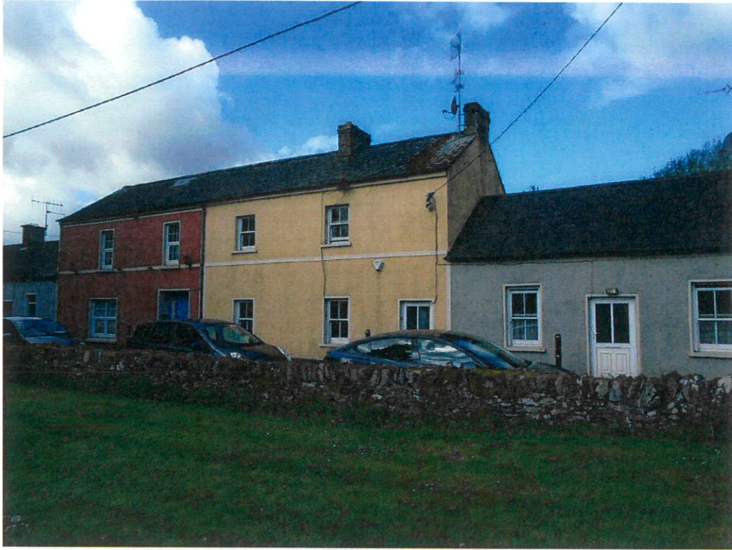
EXISTING EAST (FRONT) ELEVATION No.'s 7 - 9
