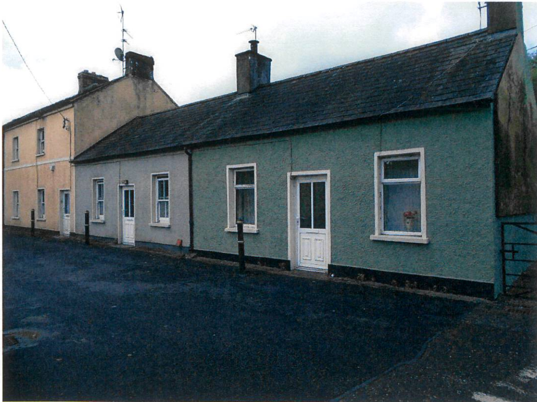
EXISTING EAST (FRONT) ELEVATION No.'s 8 - 10
