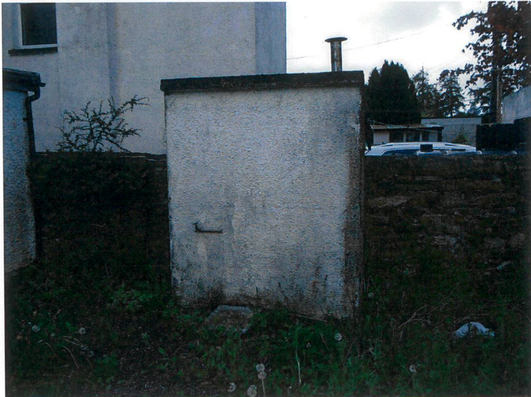
EXISTING TOILET ENCLOSURE TO BE DEMOLISHED
