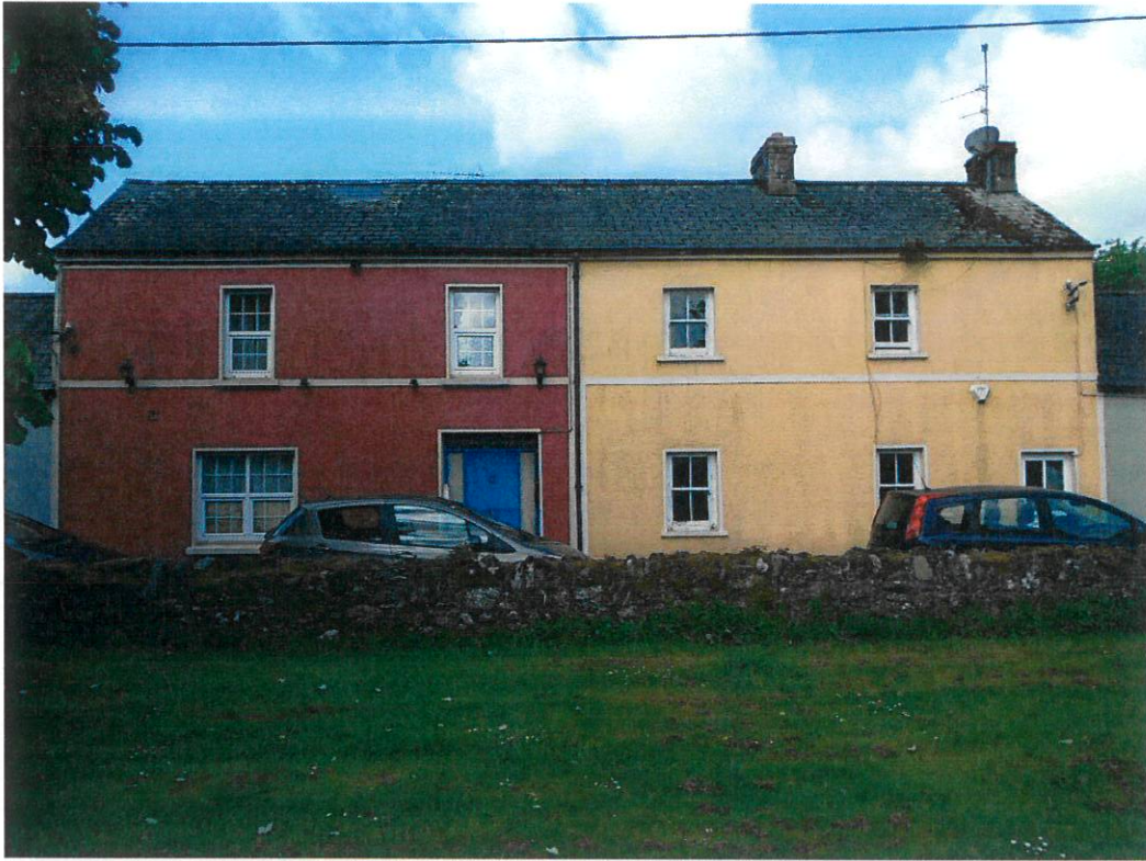
EXISTING EAST (FRONT) ELEVATION No.'s 8 & 9
