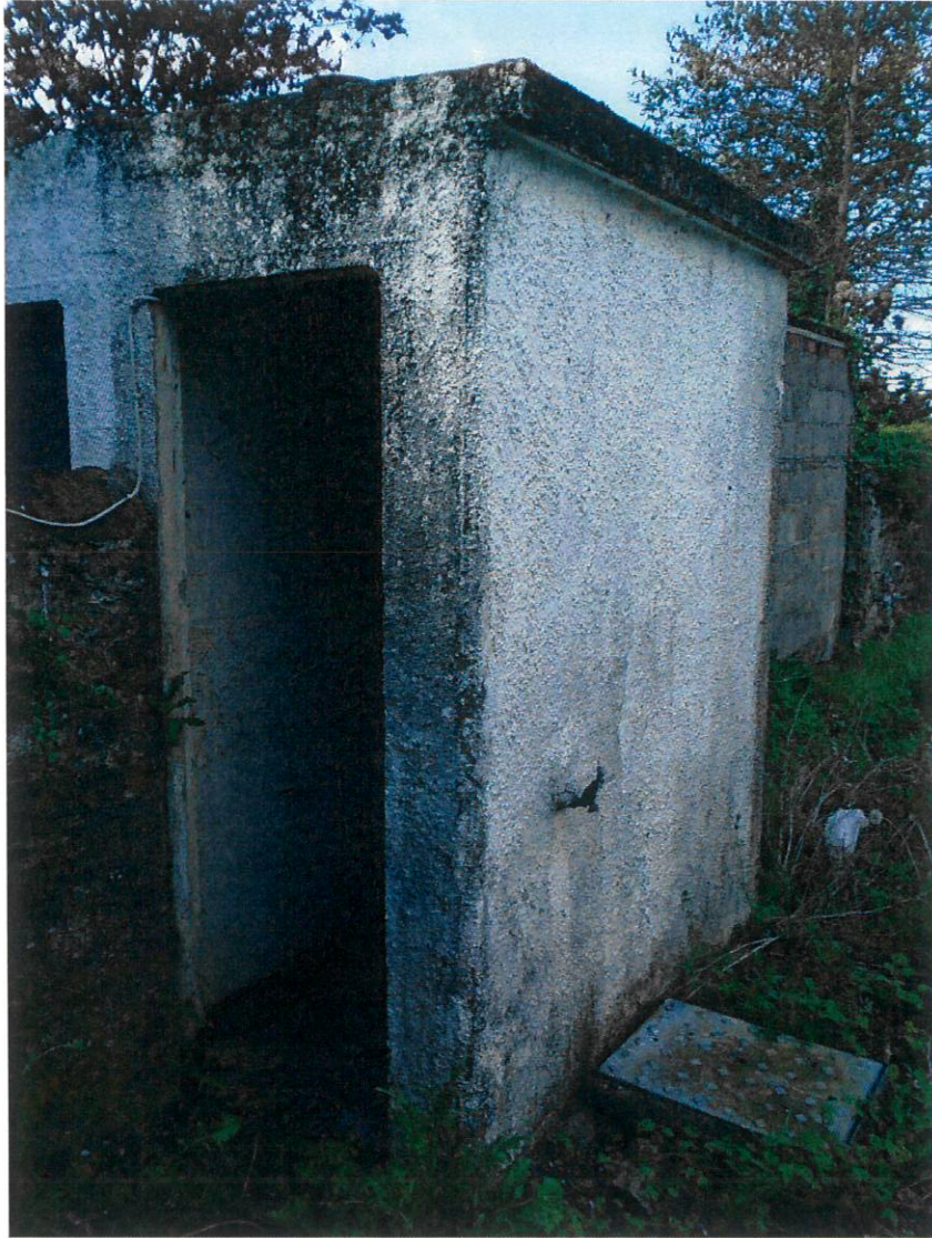
EXISTING TOILET ENCLOSURE TO BE DEMOLISHED
