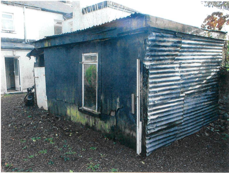
ORIGINAL OUTBUILDING (DEMOLISHED CIRCA NOVEMBER 2020)
