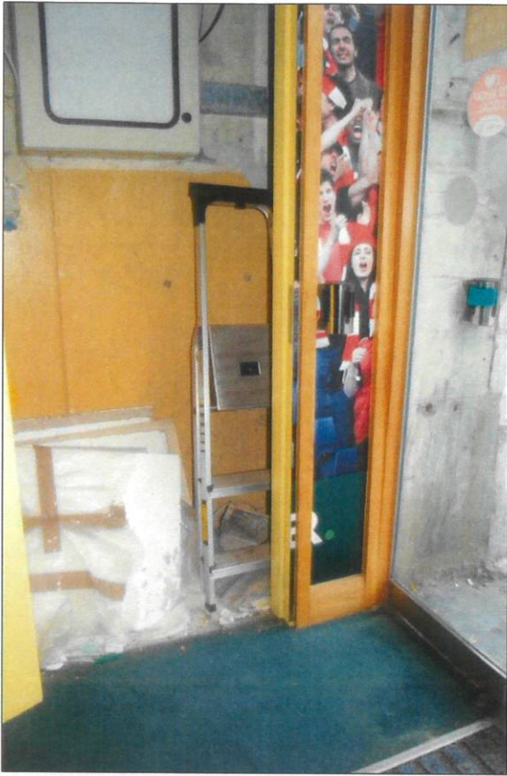
Plate 8: Modern studwork to inside
