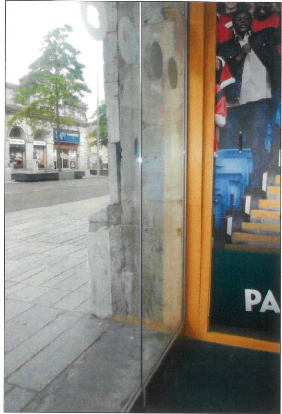
Plate 9: Glass panel fitted inside stone facade
