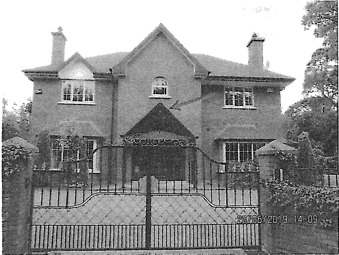
Subject dwelling to which works proposed Supported canopy to be removed and replaced with new flat roofed enclosed porch
