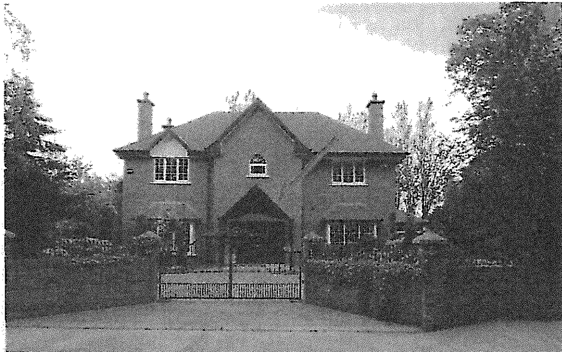
Supported canopy to be removed and replaced with new flat roofed enclosed porch
