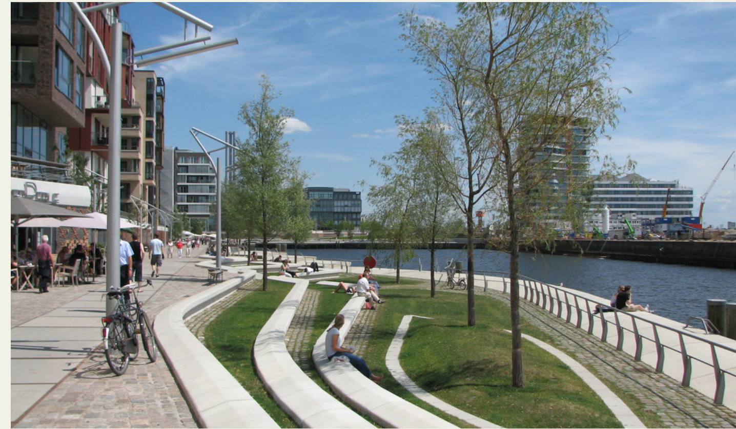
Flood defence and public amenity at Hafen City, Hamburg
