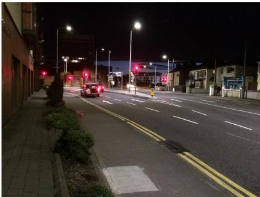
Victoria Cross after public lighting upgrade to LED
