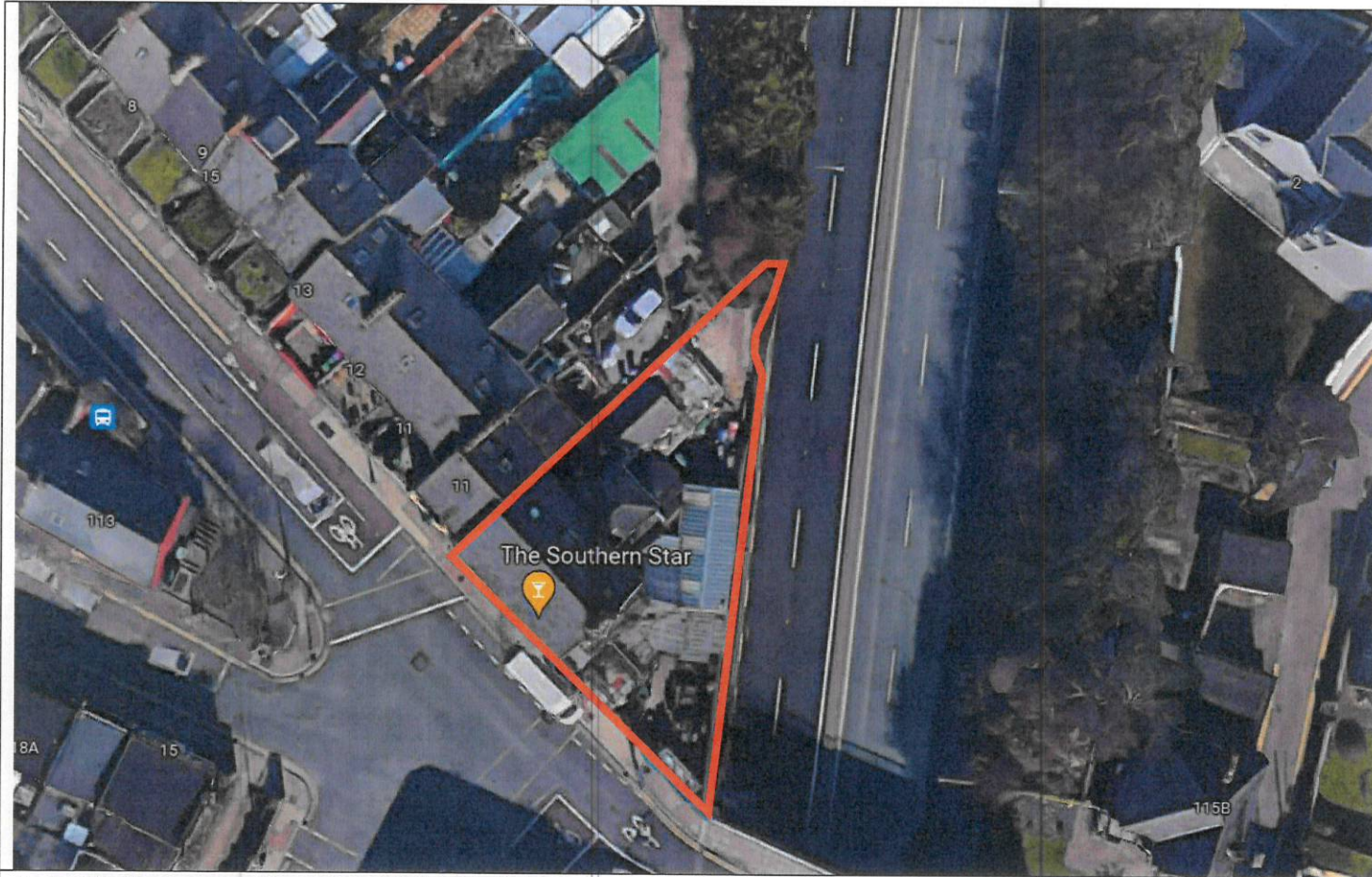
Aerial Photo showing the extent of the roofed structures within the Garden Bar prior to the recent improvements
